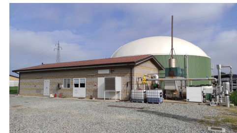
Ancillary services and digestates storage tank
